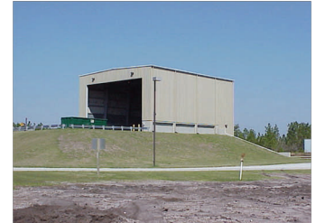
Grantsboro Transfer Station
