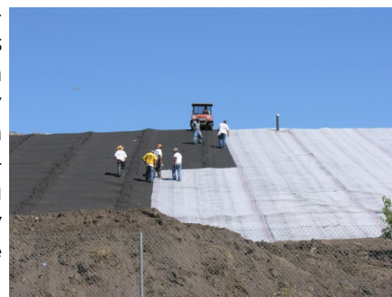
Glover Construction Crew installing liner materials
